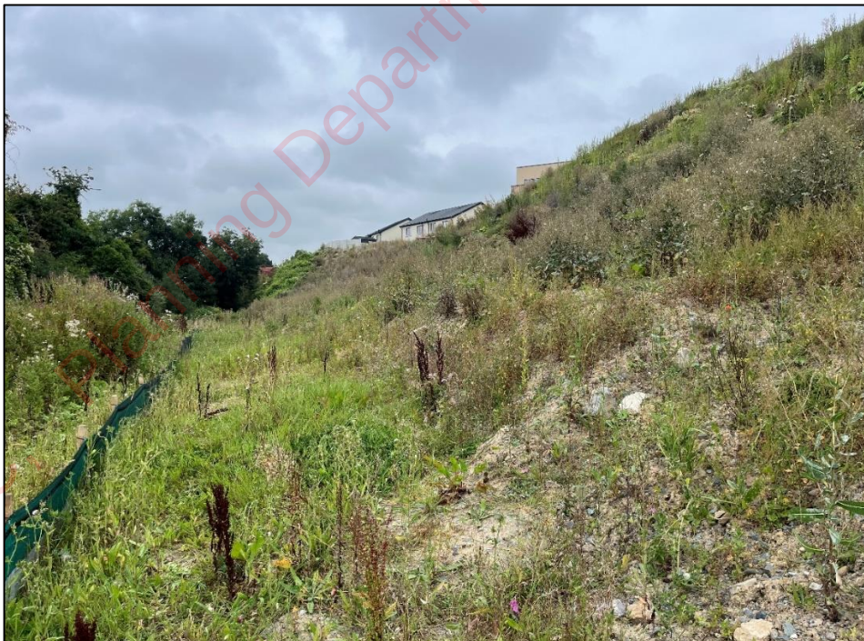
Plate 2.1 Phase 3 site looking north along the Mell Stream. Stockpiled soil is on the right hand side of the photo, and the silt fence on the left indicates the location of the Mell Stream. (Photo taken August 2025).
